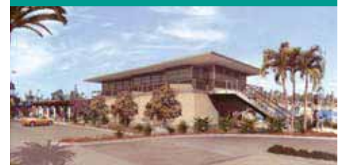
Construction will soon begin on the Yacht Club/Marina Support Building Project that extends from the west end of City Hall to past the city’s Tennis Center on Glorietta Boulevard.
