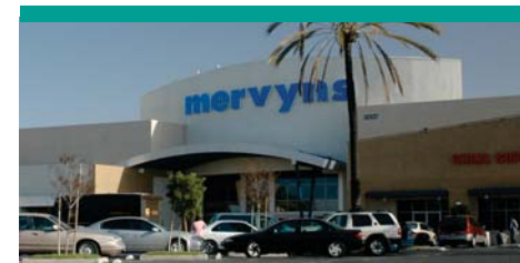
Highland Avenue is the third-largest generator of sales tax revenues for National City and includes the newly opened Mervyns store.
